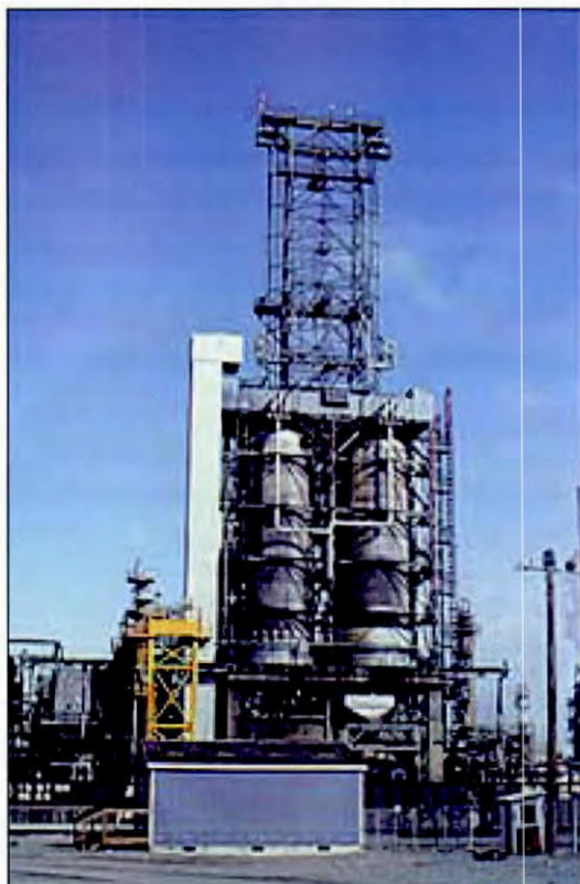
Figure A-1. Shell Delayed Coking Unit Puget Sound Refinery
